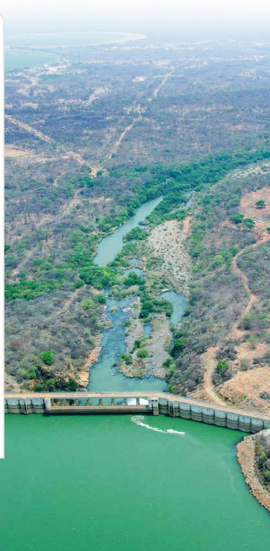
East Range Mafuro Farm in Kwekwe draws water from the Sebakwe Dam located less than 10 kilometers from this farm for its pasture irrigation
